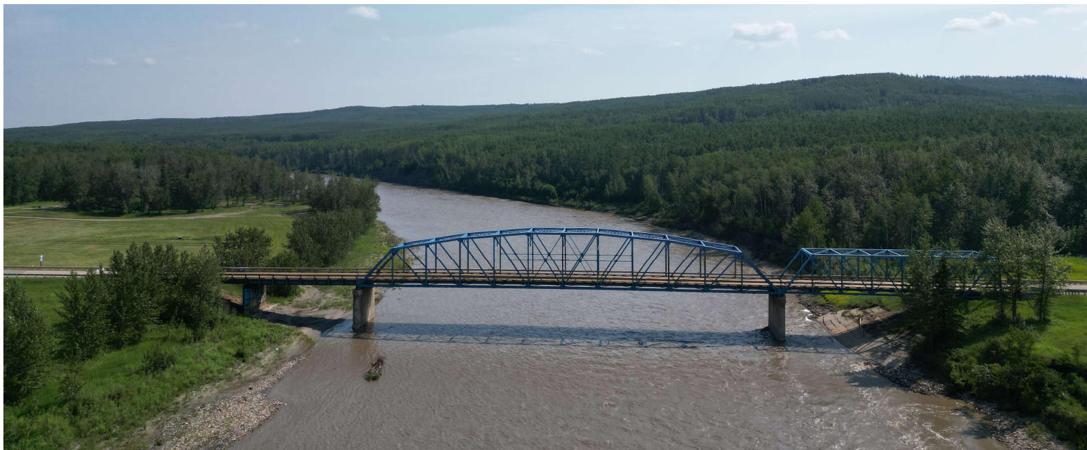
Highway 744 Smoky River Bridge Looking South
