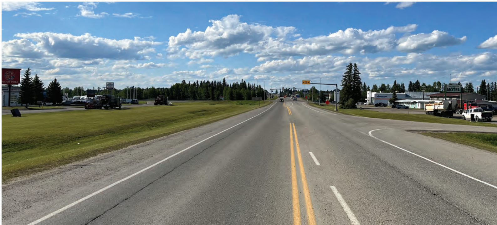
Highway 11 Looking North towards 42 Avenue
