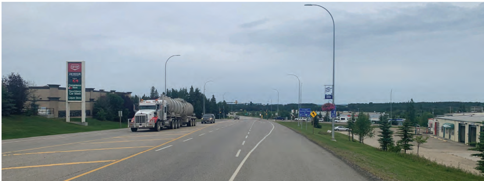
Highway 11 Looking North towards 53 Avenue
