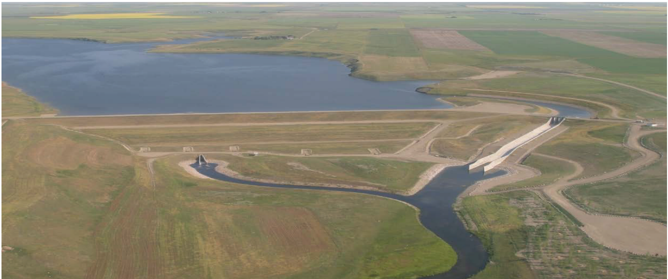
Figure 1.0 Twin Valley Reservoir Earthen Dam
